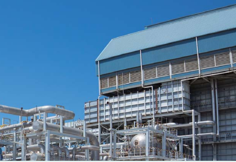
◀ Hainan Phase II methanol plant
